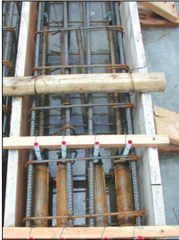
Grout sleeve connection between stacked panels.
