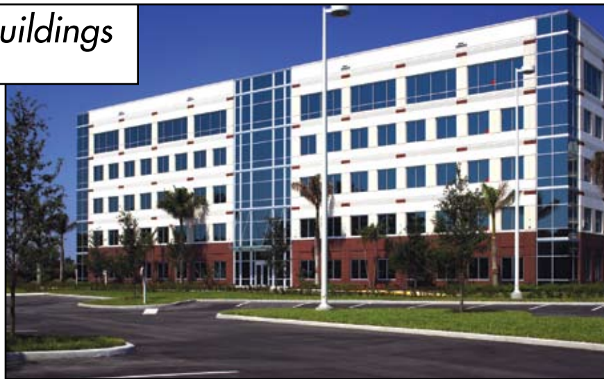
Five-story tilt-up building. Courtesy of Tilt-Up Concrete Association, ©John Gillan Photography.
