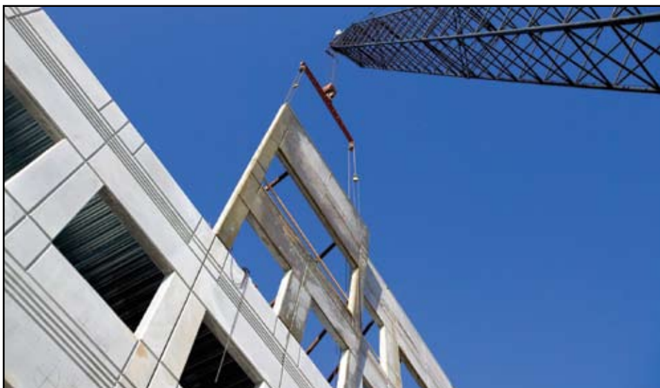
Second tier tilt-up panel lifted into place.
